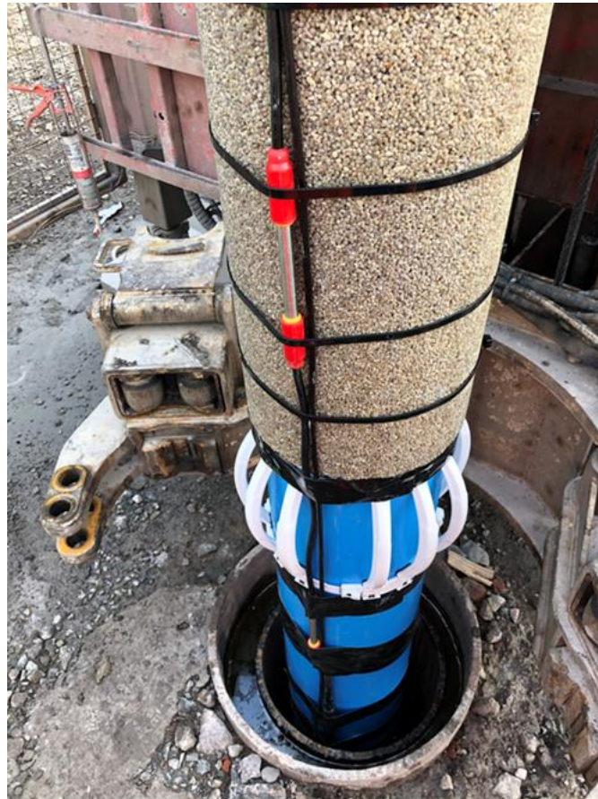
Figure 21. Installation of DTS (thin black) and ERT cables (red electrode) in a mine water geothermal research borehole (Monaghan et al. 2021)
